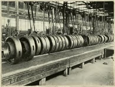
Photo from Hart-Parr Company MAKING STEEL WHEELS FOR ARTILLERY TRUCKS
