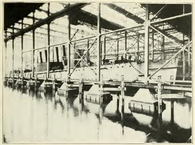
Photo from Bureau of Construction and Repair, U. S. N. BUILDING DESTROYER IN COVERED SLIP AT SQUANTUM
